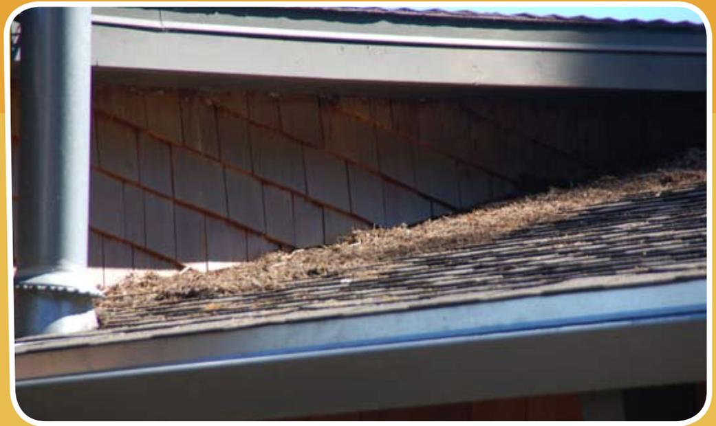
*Accumulated pine needles on this complex roof could allow embers to ignite roofing materials.*
