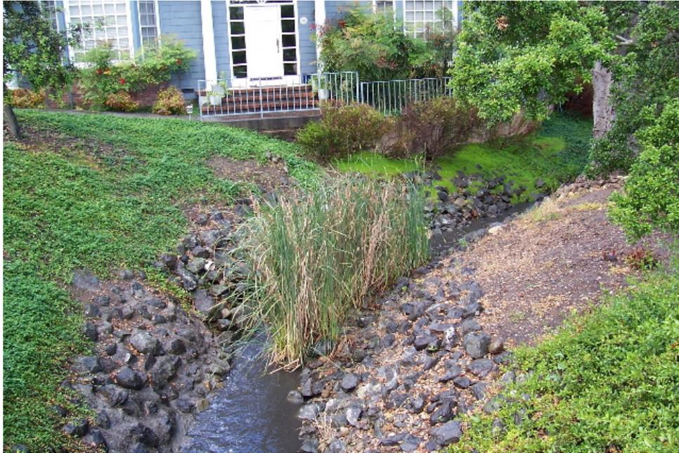
**Figure 3.** Bank stabilization installed to protect single-family residence, Menlo Park (Activity 1).
