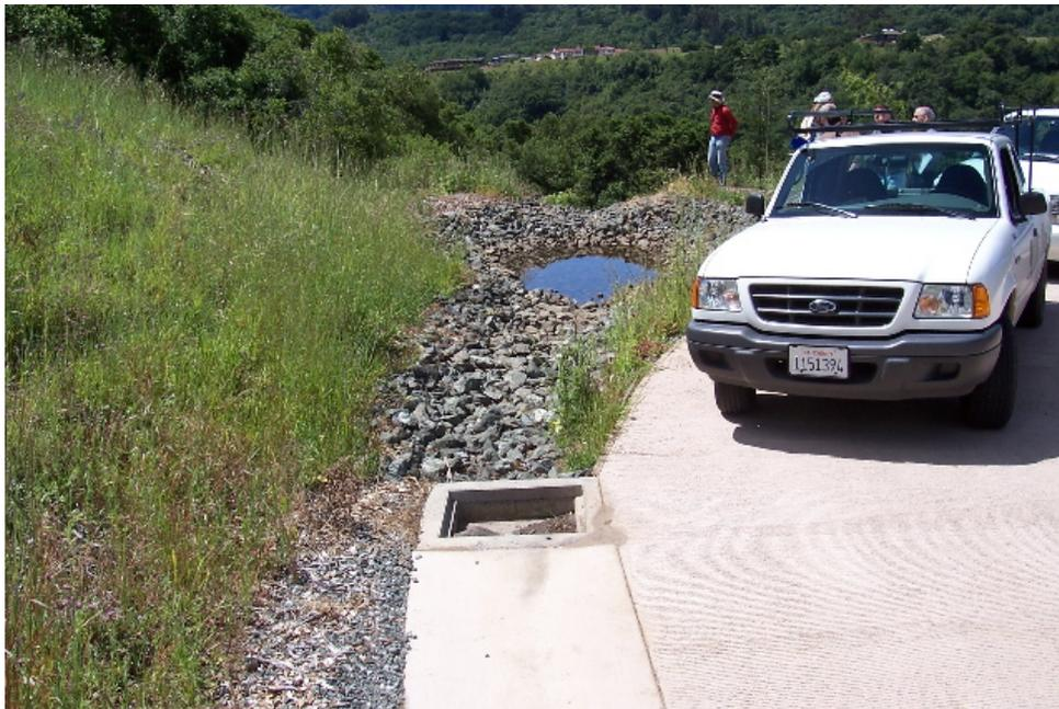
**Figure 19.** Sediment trap along access road to Los Trancos Road subdivision.
