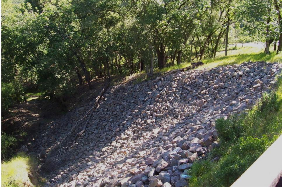
**Figure 12.** Slope protection applied to unstable area along access road, Blue Oaks subdivision, Portola Valley.
