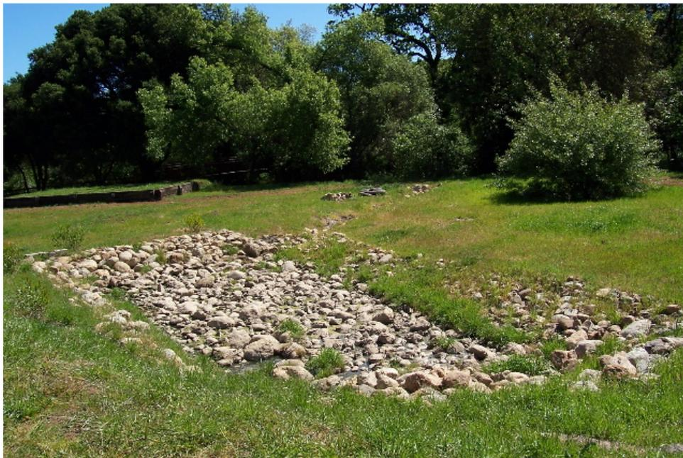
**Figure 9.** Rock-lined detention basin and drain, Los Trancos Creek, Portola Valley. This type of storm water management practice is commonly applied to new developments in the watershed by all jurisdictions. It is effective in reducing impacts on peak flows as well as reducing non-point source pollution.
