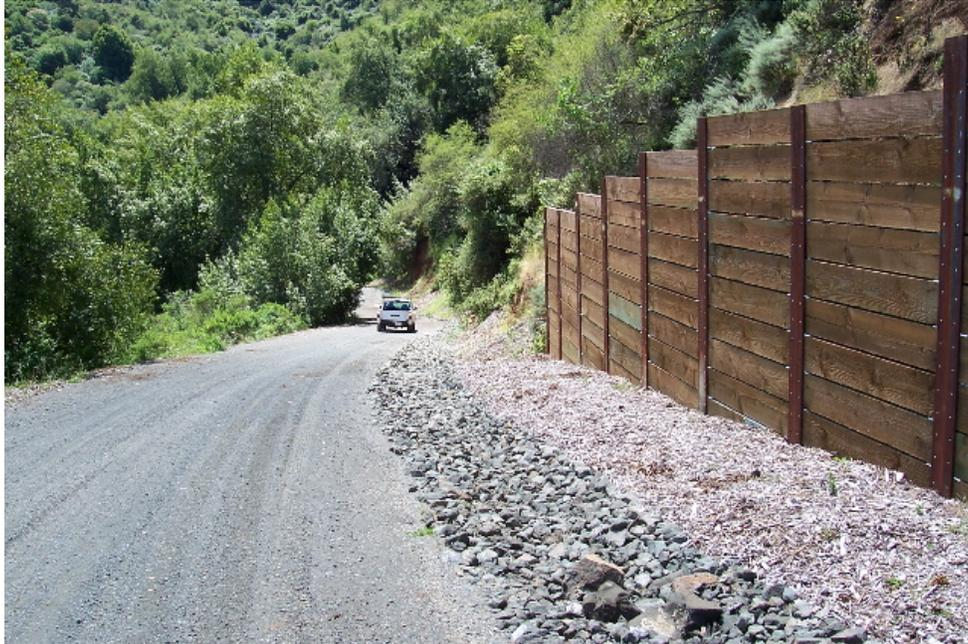
**Figure 20.** Rock-lined inboard ditch along emergency access road, Los Trancos Road subdivision. This treatment pre-dated the subdivision.
