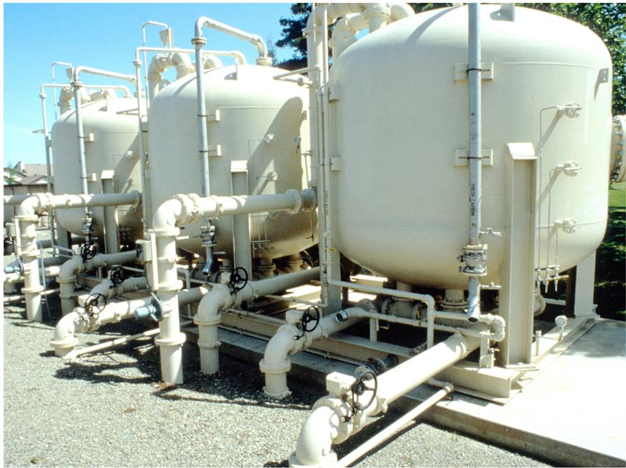
*A well-thought-out contingency plan includes provisions for installing treatment systems on water sources that have become contaminated. These Calgon granular activated carbon filters remove dibenzochlorophenol, commonly known as DBCP, at a groundwater well serving residents of Lodi, California.*
