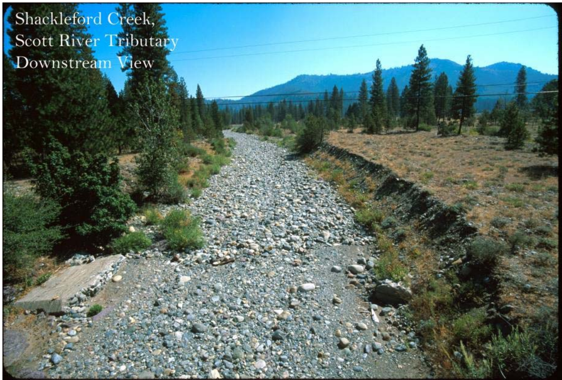
Figure 10. Shackelford Creek looking downstream at a bridge over a middle reach showing complete loss of flow due to diversion. Photo from KRIS V 3.0 taken by Michael Hentz.
