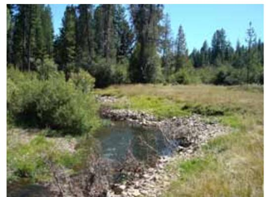
In some areas, channel dimensions were reduced by adding cobble to the riffles to raise the base elevation of the creek. Trees and rock were placed along the outward bends to stabilize the banks.
