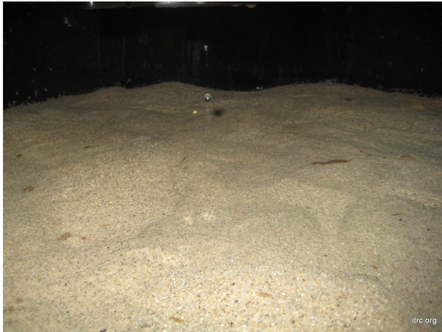
Figure 32. Arkal AGF-48" media bed after media cleaning
