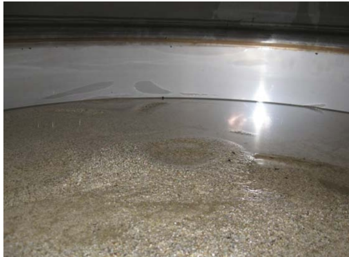
Figure 34. Lakos media bed after media cleaning
