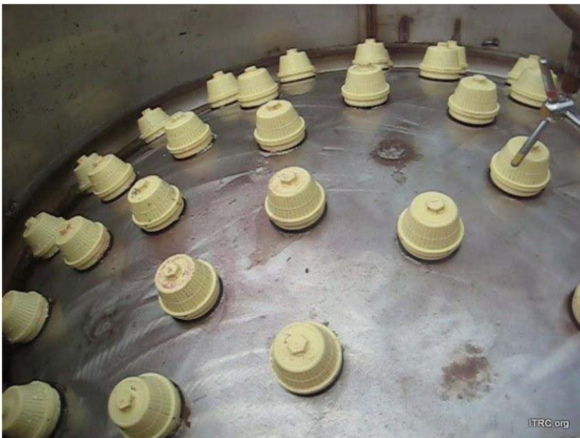
Figure 10. Waterman Dome underdrain. The pods are at different heights, due to the shape of the inverted dome. Photo shows at least 3 locations where pods were expected to be found but were not installed.
