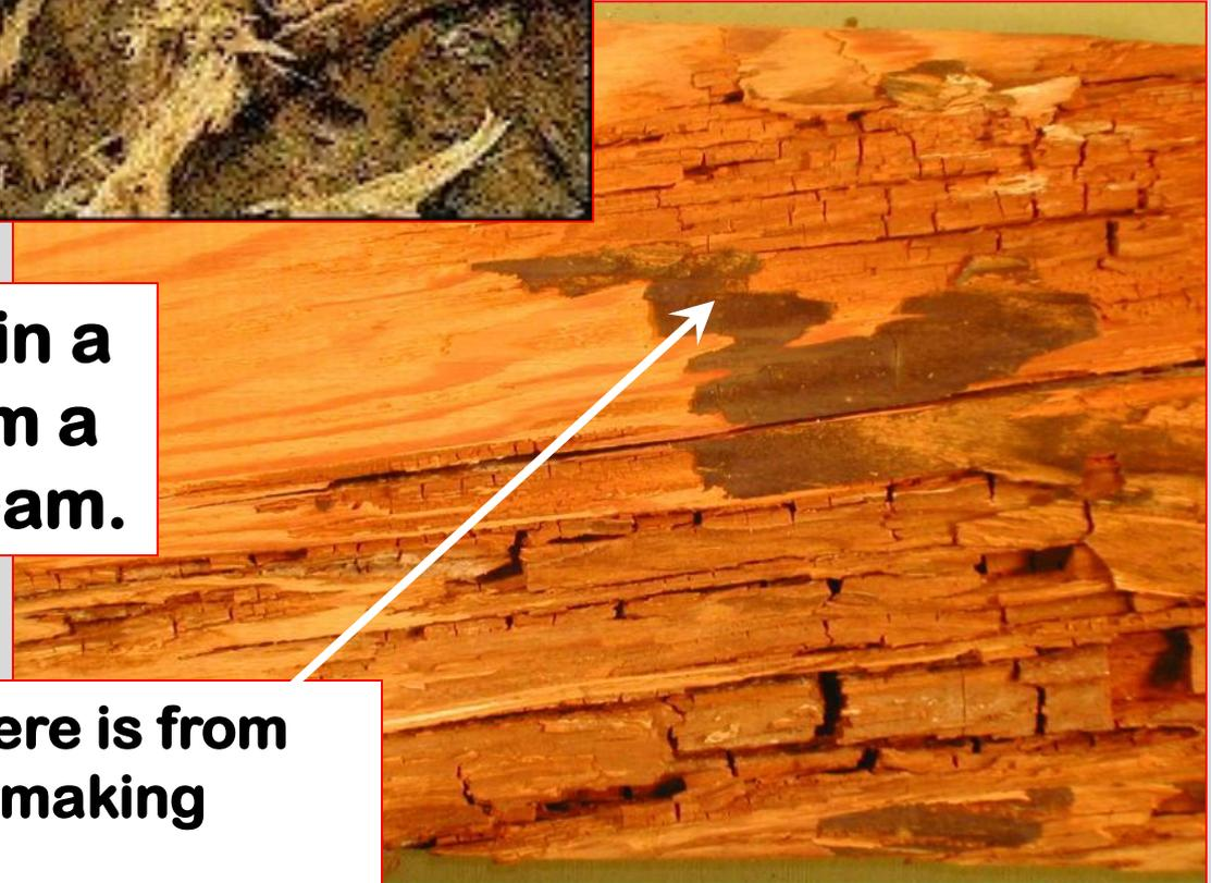
**This reddish color shown here is from the adhesive (glue) used in making glued-laminated beams.**
