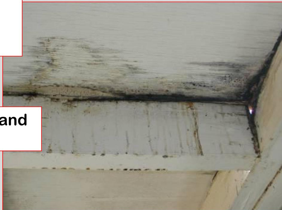
For both “*Meruliporia*” and “non-*Meruliporia*” damage you are eliminating the source of water, and replacing damaged wood. With *Meruliporia*, in order to eliminate the source of water you have to sever all rhizomorphs entering the building, and modify the construction detail to prevent entry of other rhizomorphs in the future.
