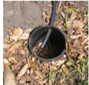
Figure 3 - An example of a 'mulch shield' (source: [greywateraction.org](http://greywateraction.org)).
