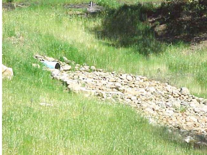
Figure 2. Culvert draining into a rock dissipater
