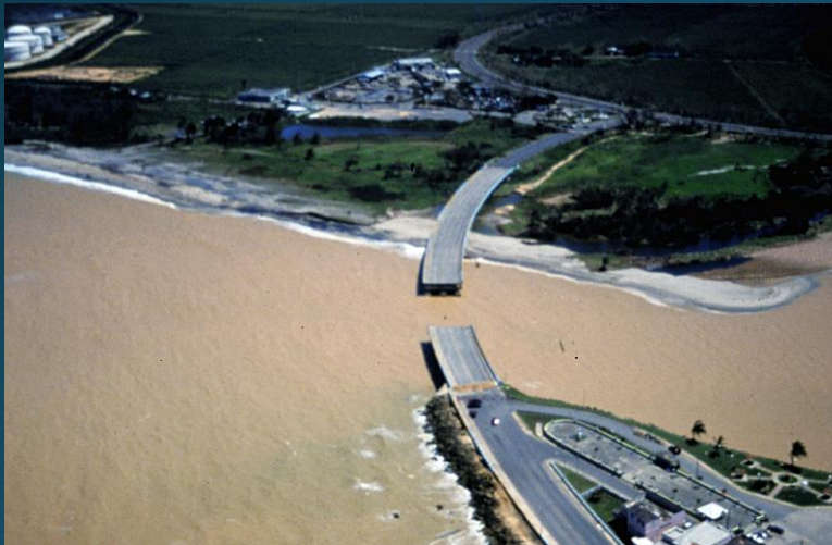
Flood damage & sediment transport, Rio Grande de Arecibo, after Hurricane Georges
