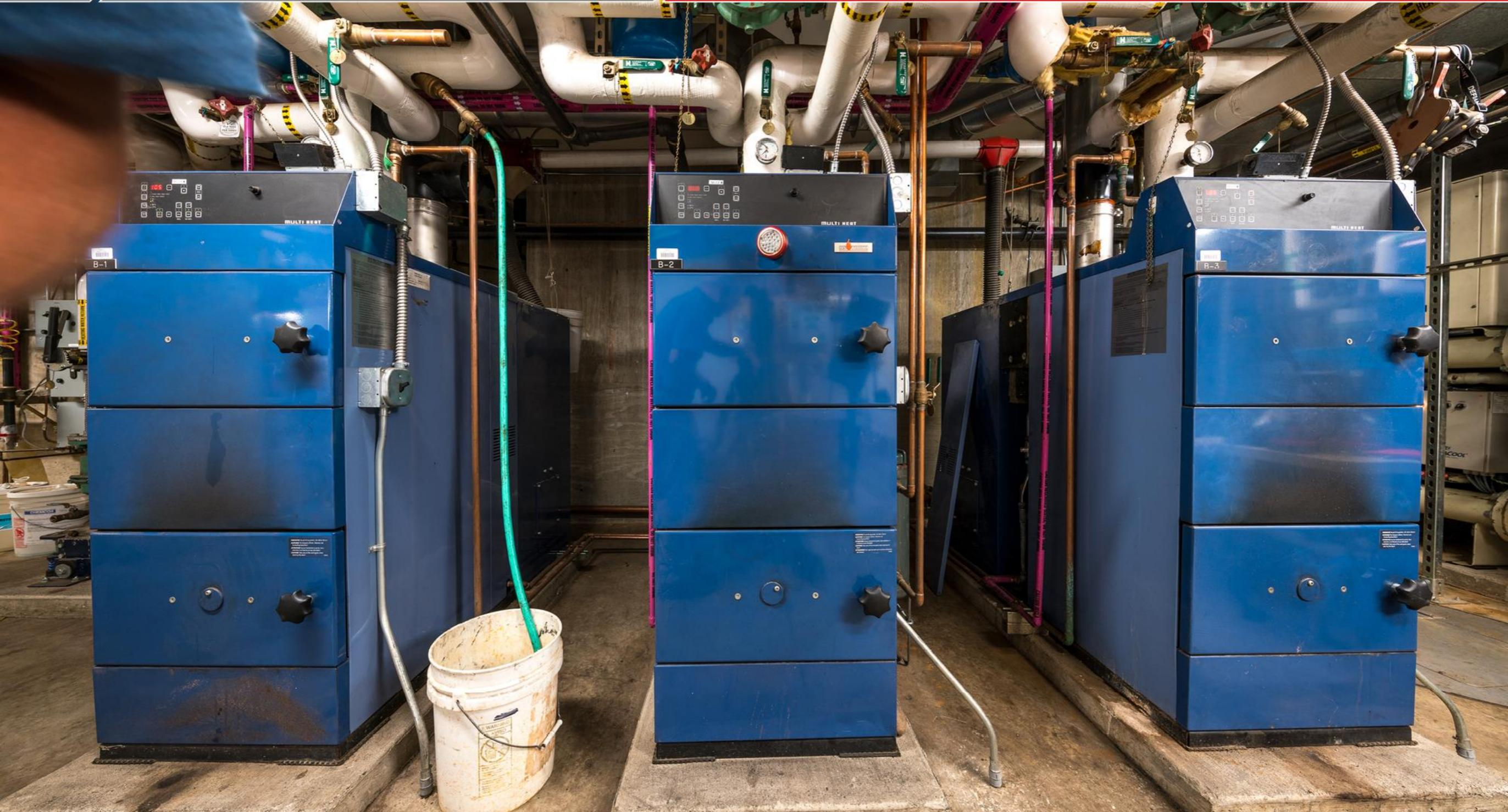
**Boiler System:** approximately 280 sq. ft. (20' x 14') of the 1,500-square foot mechanical equipment room is dedicated to the biomass boiler system. The system is made up of three TARM 136,500 Btu/h wood pellet boilers. Each boiler has an internal pellet storage bin that is semi-automatically filled from the large pellet silo outside.
