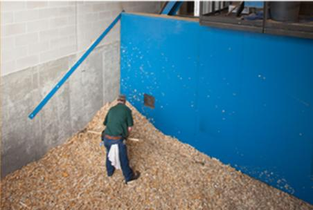
**Where will you store the biomass fuel?** Most biomass facilities store between a week of fuel and a whole heating season of fuel. That fuel is usually stored next to a biomass boiler to make supplying the fuel easy. Add a rectangle to your site diagram of the dimensions specified in the Biomass Design Parameters. Label this square something like "Future Biomass Storage Facility."
