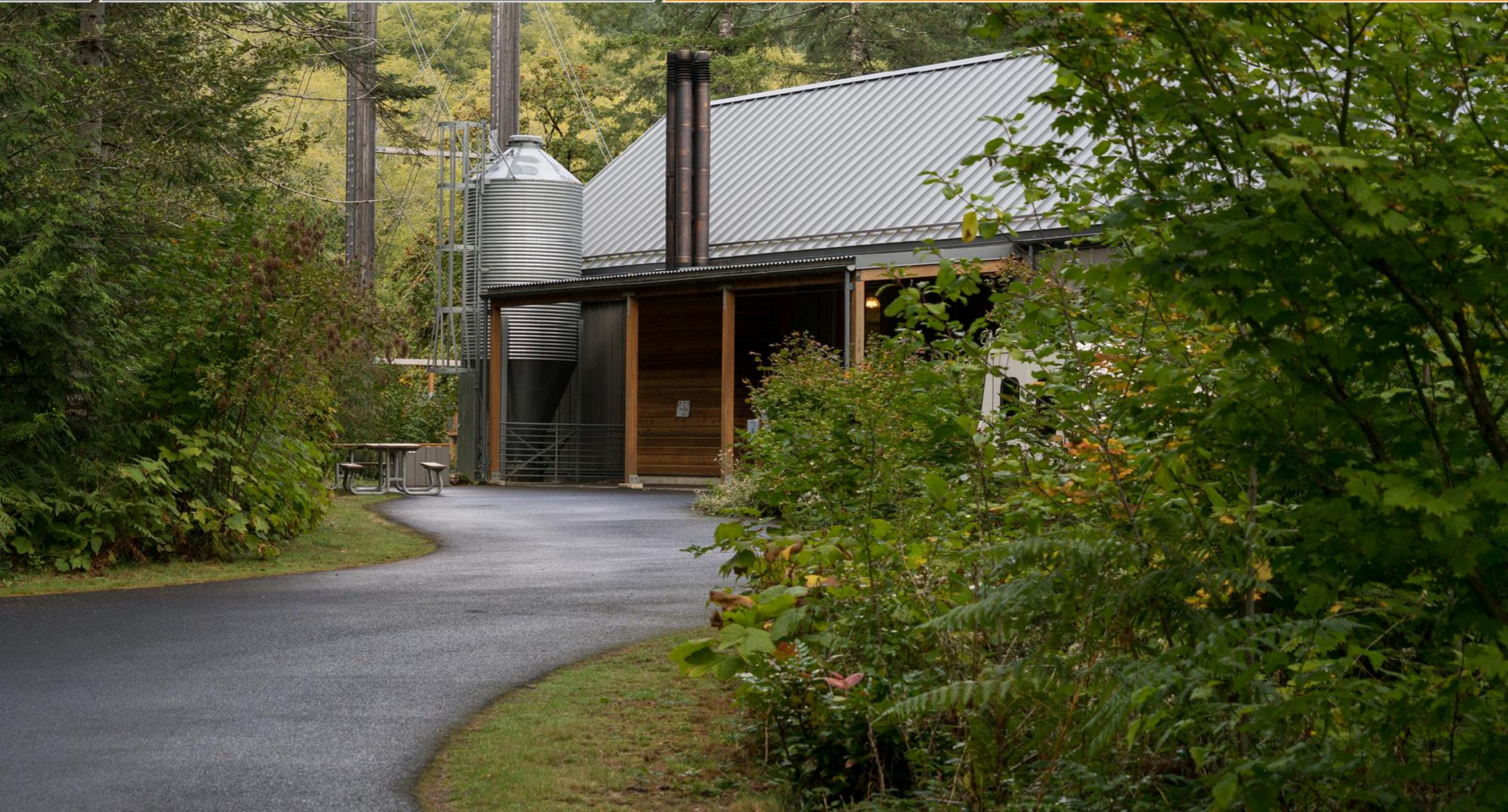
**Storage:** Approximately 64 sq. ft. (8' x 8') are needed for the 7' diameter, 24' tall, 10-ton grain silo used to store enough pellets to heat the building for a typical winter season. The architects incorporated the agricultural silo into the building's design helping reinforce the theme of a working sawmill.
