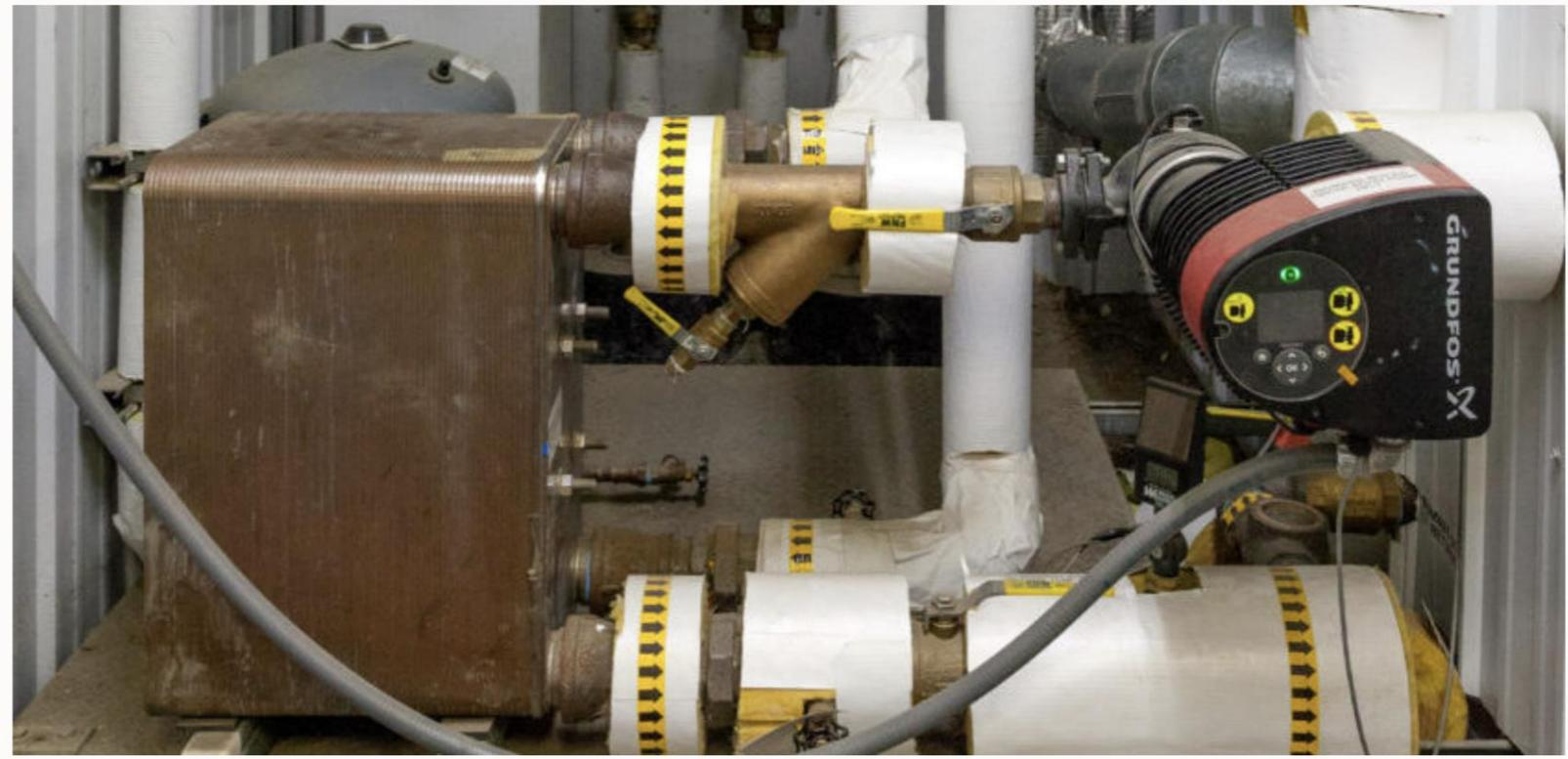
Your HVAC system is compatible with 180-degree hotwater loop from the biomass boiler.
