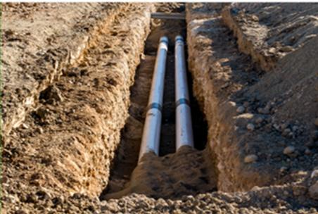
**How will you connect your boiler to your building?** Heat distribution piping is expensive – especially if it needs to be buried – so the closer the boiler building is to your new building, the better. Add a line or path to your site diagram connecting the biomass boiler facility to your building's mechanical room. Label this line something like "Future Biomass distribution pipe."
