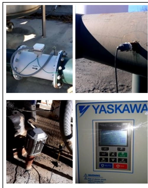
Figure 3. Magnetic flow meter (upper left), pressure transducer (upper right), acoustic groundwater level sensor (lower left), and VFD digital control panel (lower right).
