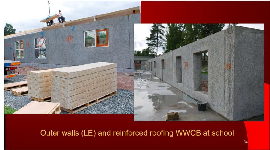
Outer walls (LE) and reinforced roofing WWCB at school
