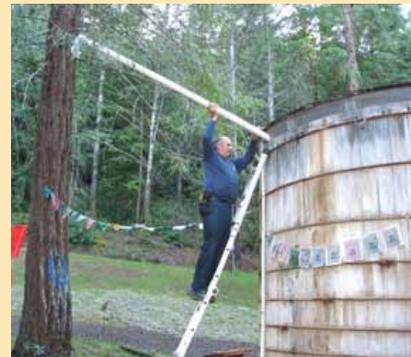
If your existing system is not sufficient or adaptable, consider purchasing a tank solely for fire protection. Place the tank at least 80 feet above the house, or as high as is practically possible. Use at least a 2" water line, and up to a 3" line if affordable and the size of the water supply justifies the expense.
