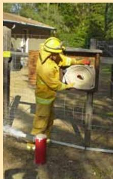
can rot quickly. Nozzles should be pre-connected to the hoses, and fire hose cabinets should be clearly marked and easy to access.
