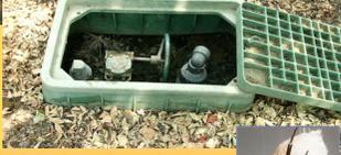
Buried vaults in the tree row protect irrigation valves, air release valves, etc. from shaker and mechanical cross-hedging, but watch out for Black Widow spiders)
