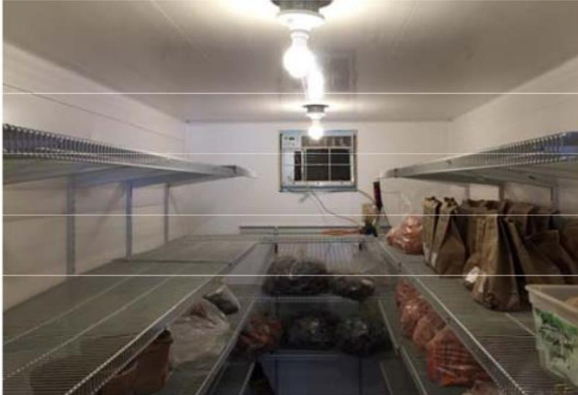
*This cooler space was finished with Trusscore PVC panels resulting in a smooth, cleanable surface.*
