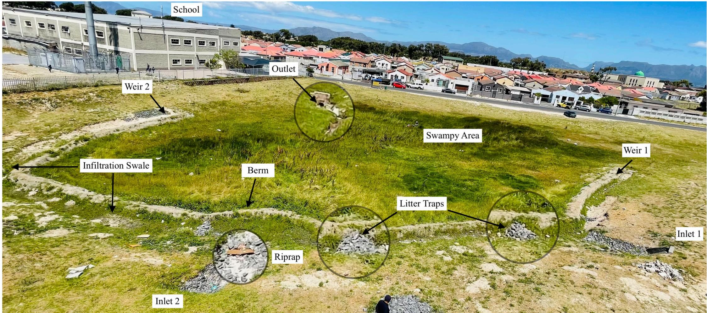
*Water enters the pond from the local stormwater drain catchment and flows into the infiltration trench in front of the inlets. This slows down the water so that it can flow through sand and the natural vegetation so that it is cleaned and filtered before reaching the outlet.*
