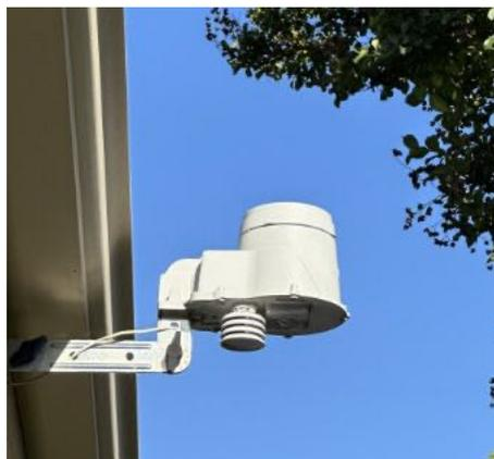
*Some smart controllers are wi-fi enabled and download weather information from the internet. Others are connected to weather sensors attached to the home, like this one.*
