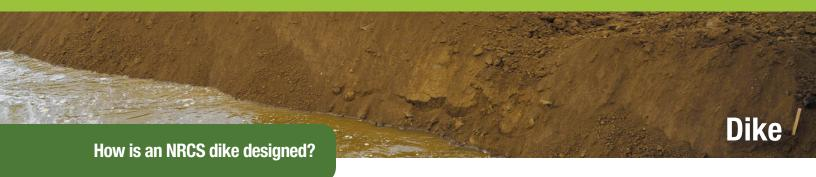
**Height**: The top of the dike is set to prevent overtopping from a storm frequency consistent with the hazard involved, but should not be less than a 25-year frequency, 24-hour duration storm. Dikes protecting major structures, homes, school buildings and high capacity roads should have enough height to prevent overtopping from a 100-year frequency 24-hour duration storm. A hydrological analysis should be completed to account for the burned acres within the watershed.
